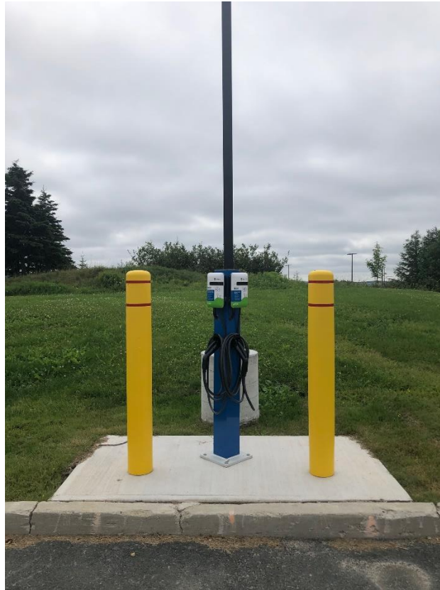
Figure 1: Duel Port Single Bollard Installation
