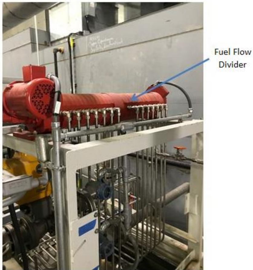
Figure 1: Fuel Flow Divider – Holyrood Gas Turbine
