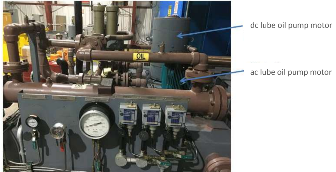
Figure 3: Lube Oil Pumps - Happy Valley Gas Turbine
