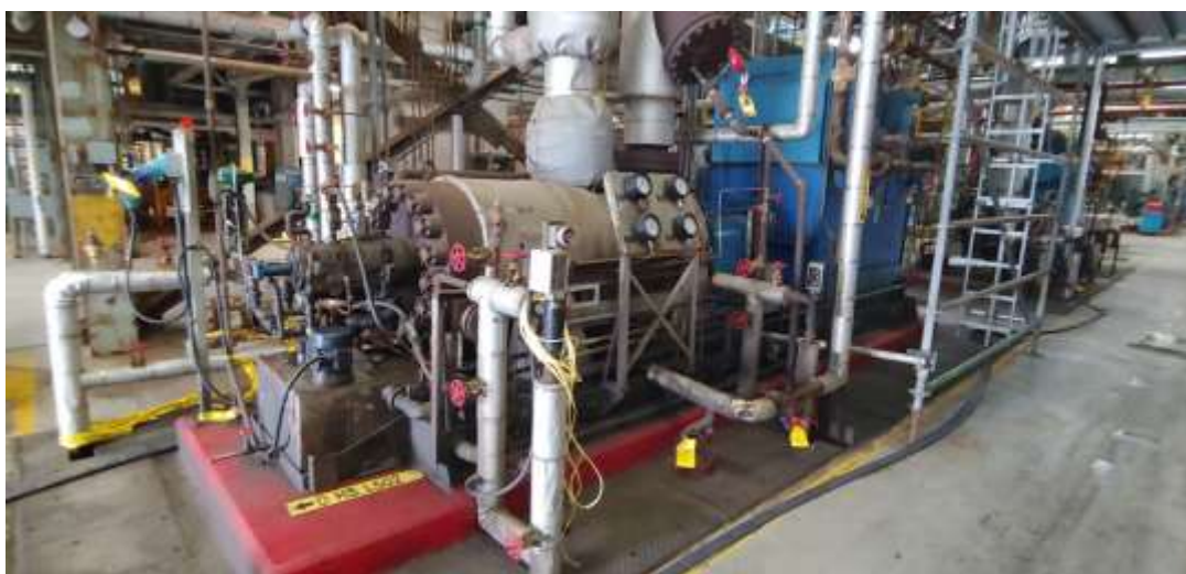
Figure 1: Unit 3 Boiler Feed Pump East
