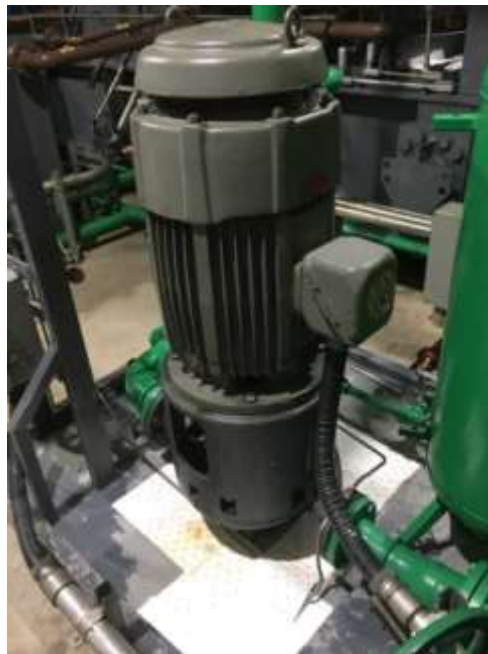
Figure 4: Glycol Pump - Happy Valley Gas Turbine
