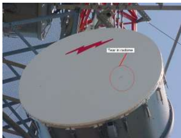
Figure 2: Tear in Radome
