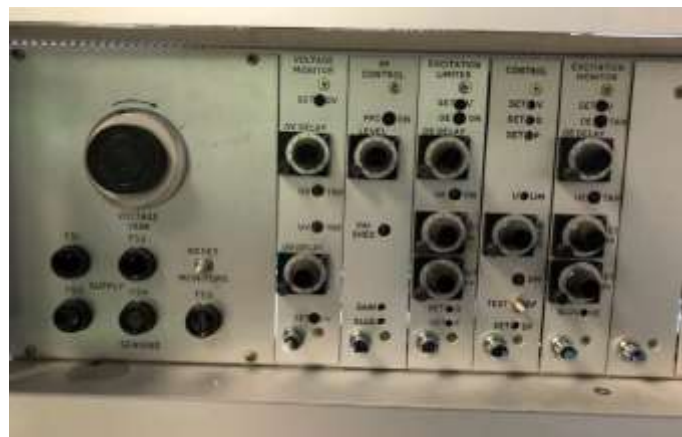
Figure 1: AVR Front Panel
